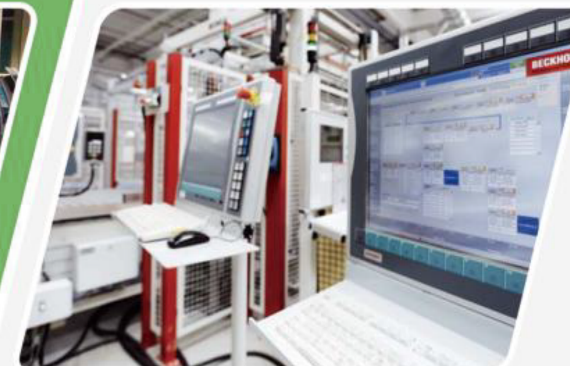
Equipment Control Terminals
